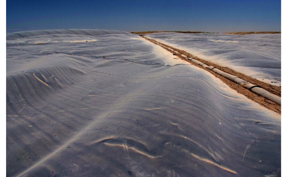
► Above: This 37-million-gallon digester extracts methane from manure in a 40-day cycle. The gas helps satisfy California’s demand for renewable energy. ► Left: David Albers, a dairyman/lawyer, created a new model for digesters and a win-win for producers, utilities, and the environment.
